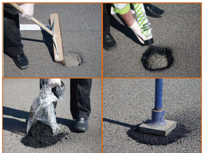
Ultracrete IRR step-by-step application guide
